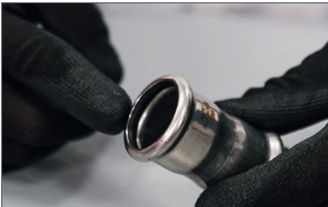
Controllo O-ring / Checking the sealing ring
